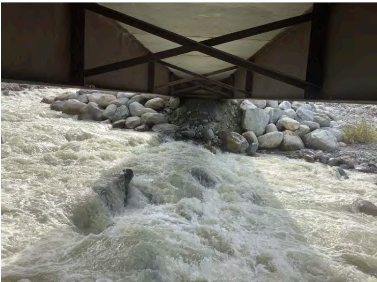
Left Bank Abutment when facing downstream
