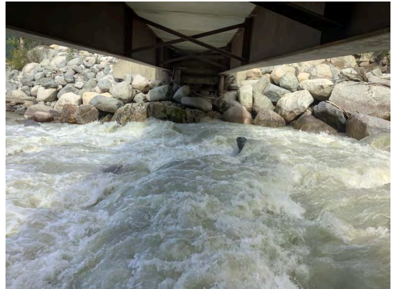
Right Bank Abutment when facing downstream
