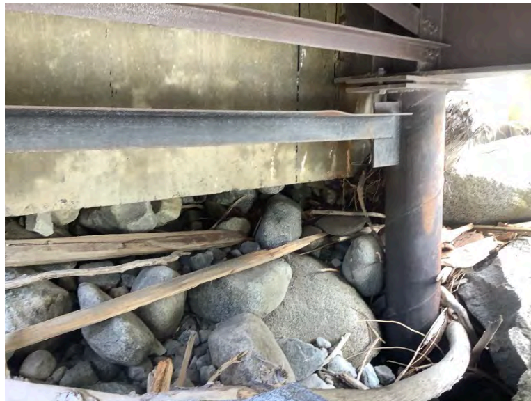
Right Bank Abutment when facing downstream
